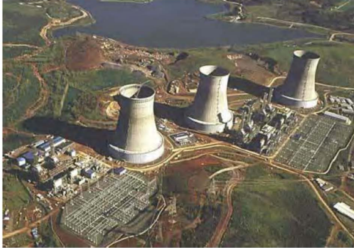
GEBZE & ADAPAZARI 3 x 777 MW e CCGP commissioned in 2002 (Turkey) EPC-Contractor: BECHTEL-ENKA JV, End-user: INTERGEN The world's largest dry cooled combined cycle power plant
