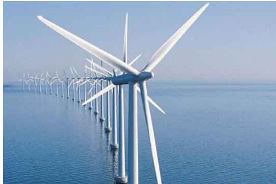
Vesta 7MW turbines, rotor D = 164 m, in an off-shore farm.
