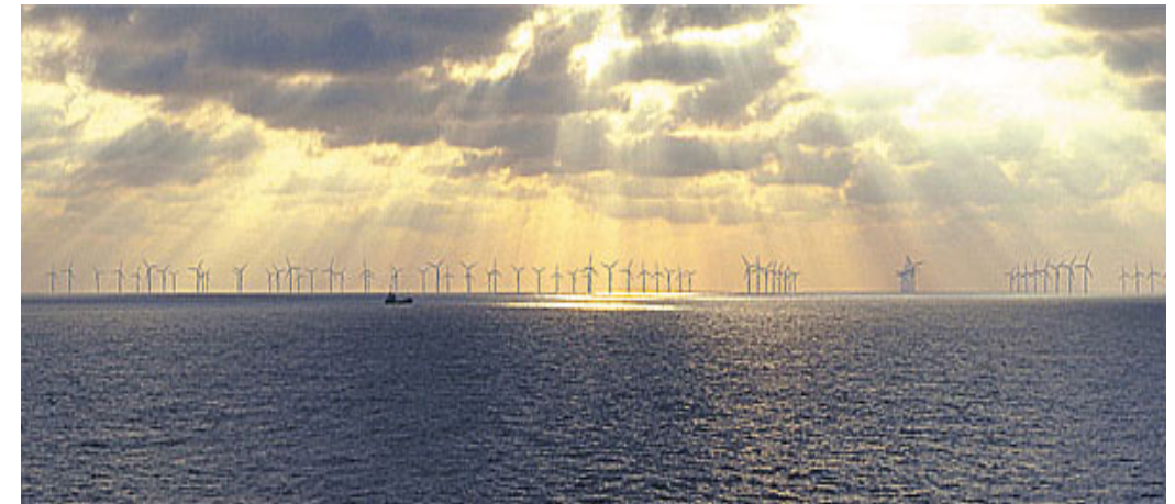
Horns Rev Wind Farm (Denmark) - Rated Power 160 MW – Water Depth 10-15m
